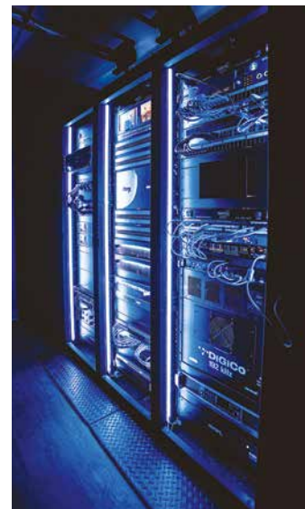
A Ross Video Ultrix-FR5 routing and AV processing platform forms the backbone of the video setup
